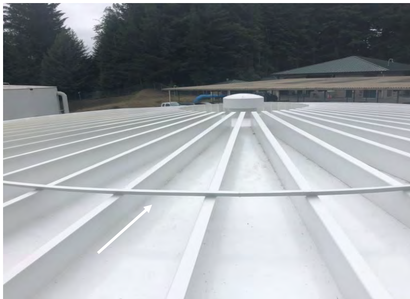
Photograph 8 – Korblex – 1 MG reservoir – Paint (white) reported to be nondetect for asbestos and lead.
