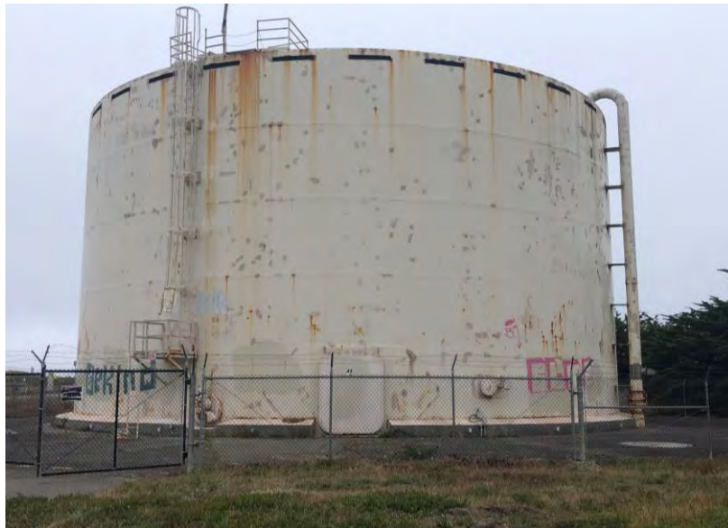
Photograph 4 – Samoa – 1 MG reservoir – View of exterior.
