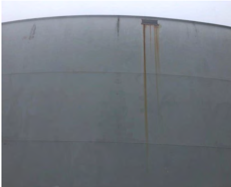
Photograph 1 – Korplex – 2 MG reservoir – View of exterior wall.
