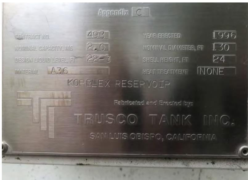
Photograph 2 – Korplex – 2 MG reservoir - Exterior at name plate.
