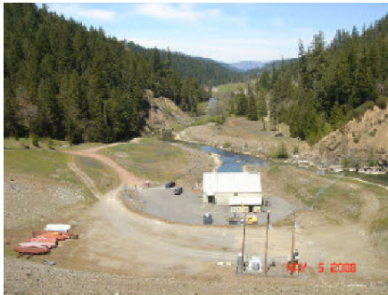
Ruth Hydro Plant View from Lower West Side Rd.
