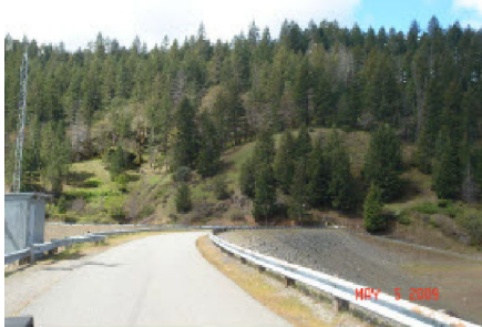
Ruth Lake top of dam above Hydro Plant
