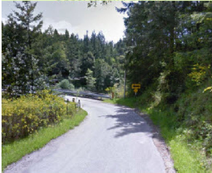
Approach to River from Butler Valley Rd.
