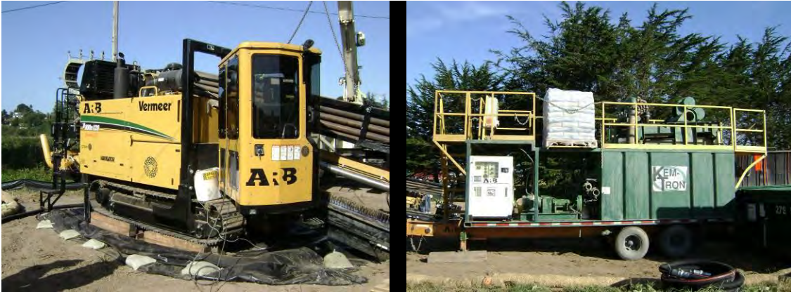
Figure 1. Drill rig placed on timber mats and plastic ground covering with silt fences in the background (left). Separation plant surrounded by straw wattles (right).
