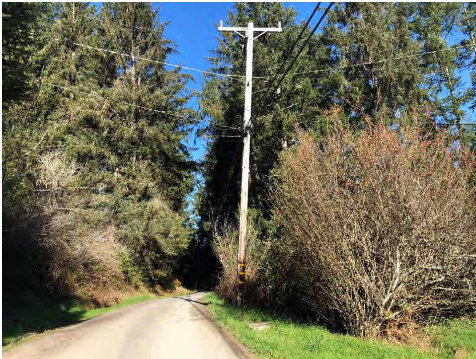
Figure D8. Facing northwest on Warren Creek Road towards the location of the modification of the existing river crossing, detail 3 sheet C-401.
