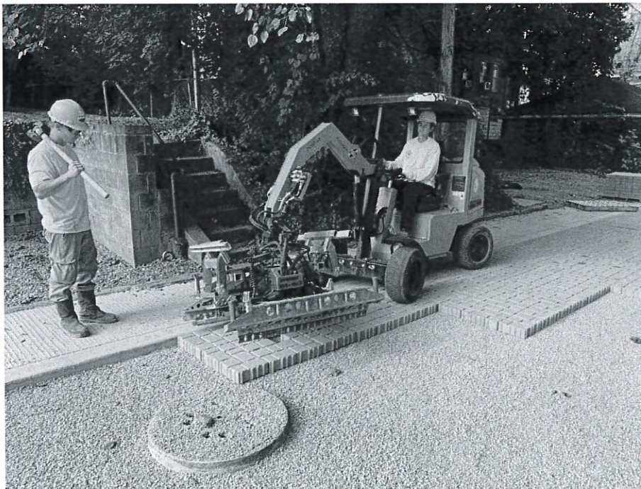
Installing permeable concrete in Pittsburgh
