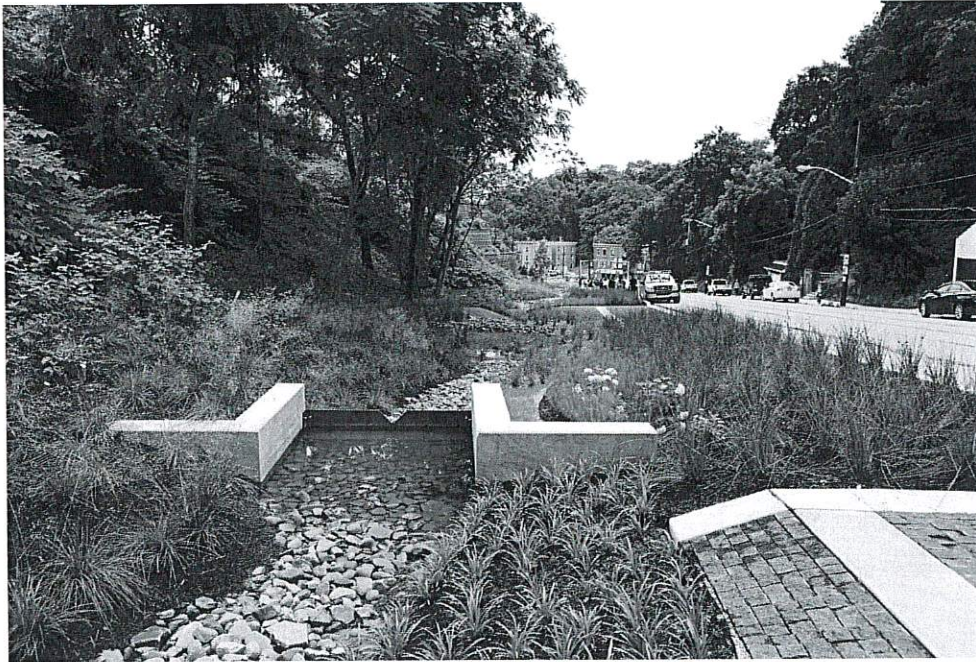
A swale collects stormwater in Pittsburgh's Hill District
