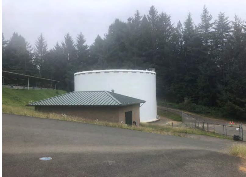
Photograph 3 – Korblex – 1 MG reservoir.
