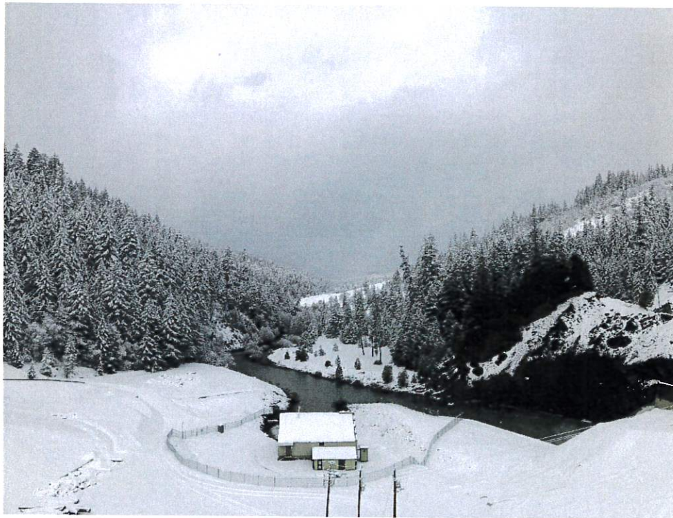
Ruth Lake Hydro Plant
