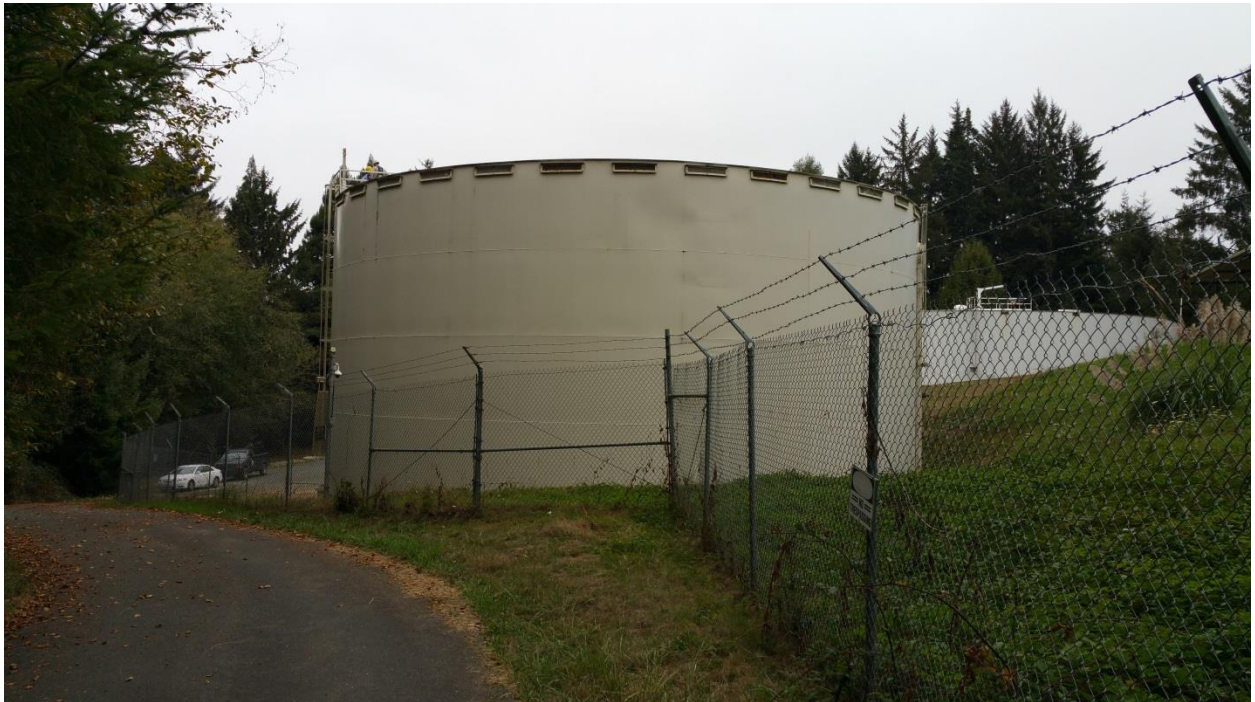
Photo 6: Tank Exterior (facing northeast)
