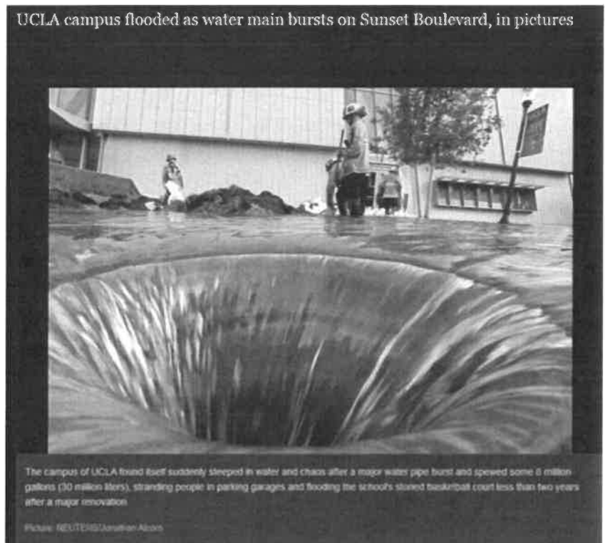
FIGURE 2 - JULY 2015 UCLA MAIN BREAK CLAIMS $13 MILLION IN FLOOD DAMAGE
