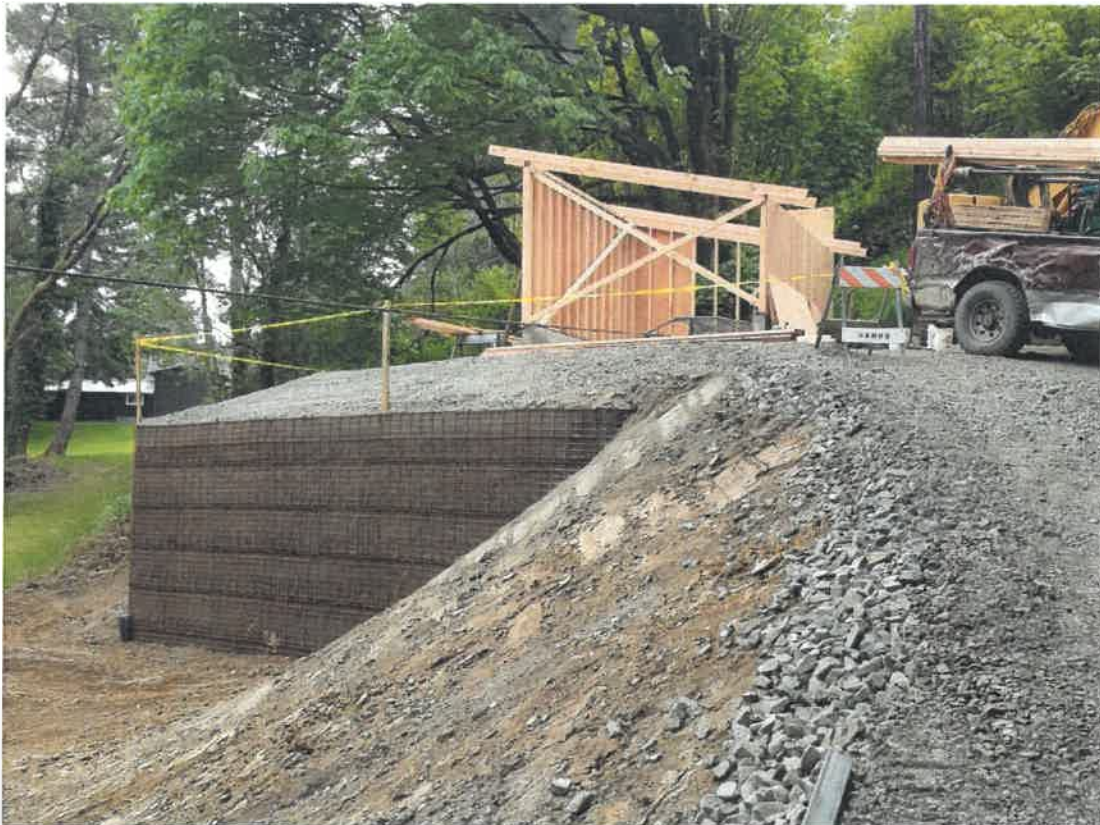
Collector 2 Cable Car Shed Rebuild
