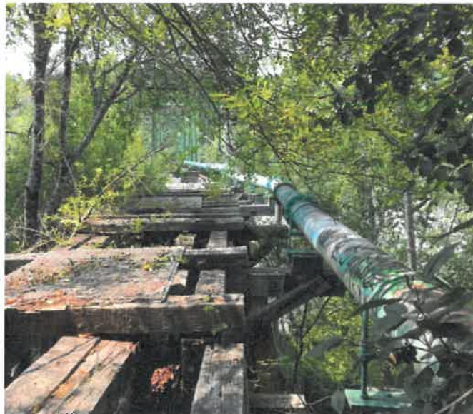
Figure 2 – HBMWD Service Area near Eureka, CA Figure 3 – Original 14" water line crossing NCRA RR bridge
