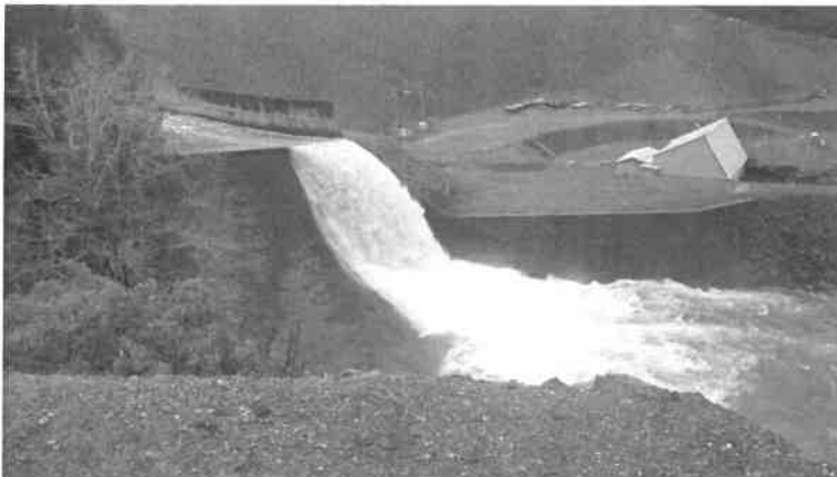
Water pushed over the Ruth Dam Spillway yesterday.
