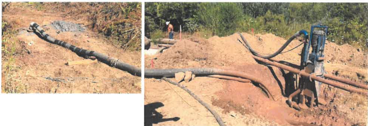
Figure 11 – “Snorkel” implemented by JCGE to contain initial inadvertent drilling fluid return
