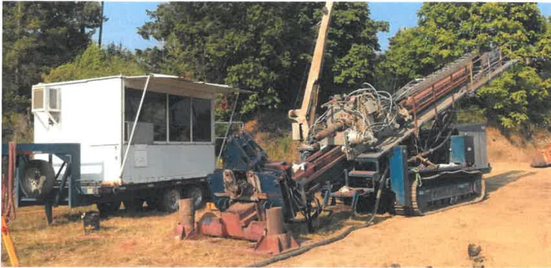
Figure 10 – JCGE's Modified American Augers DD200 drill rig
