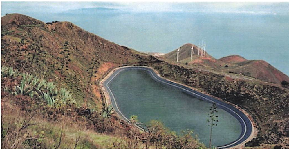
Pumped storage hydropower in the Canary Islands (Source: Idom)
