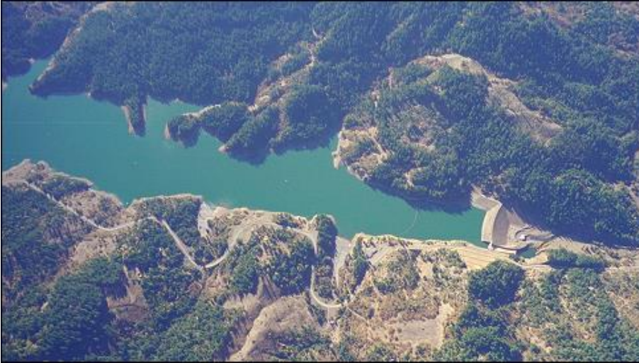
Figure 5. Aerial view of R.W. Matthews Dam and Ruth Lake.
