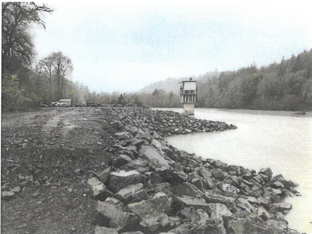
Collector 4 bank erosion work
