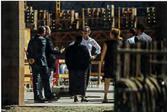
Newsom tours construction at the Antioch Brackish Water Desalination Project on Aug. 11, 2022. Photo by Martin do Nascimento, CalMatters
