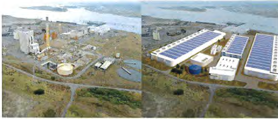
BEFORE AND AFTER Left, the degraded industrial site. Right, a visualization of the fish farm. Via County of Humboldt
